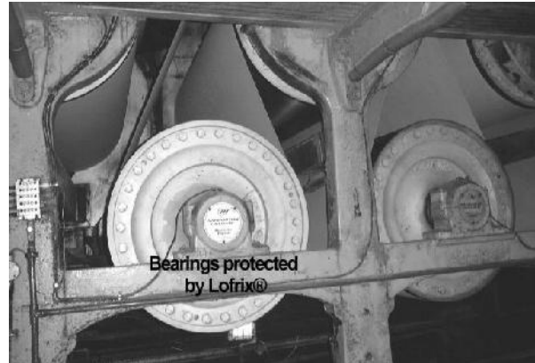
Short wave infra-red heated drying line
