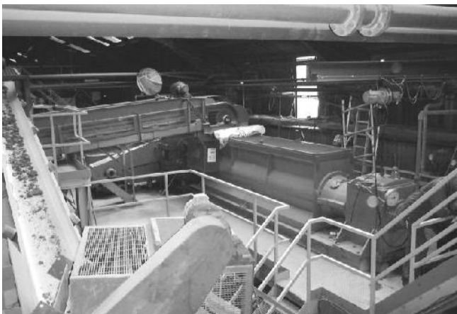
First stage clay shredder, prior to vacuum chamber and plasticising screw.
